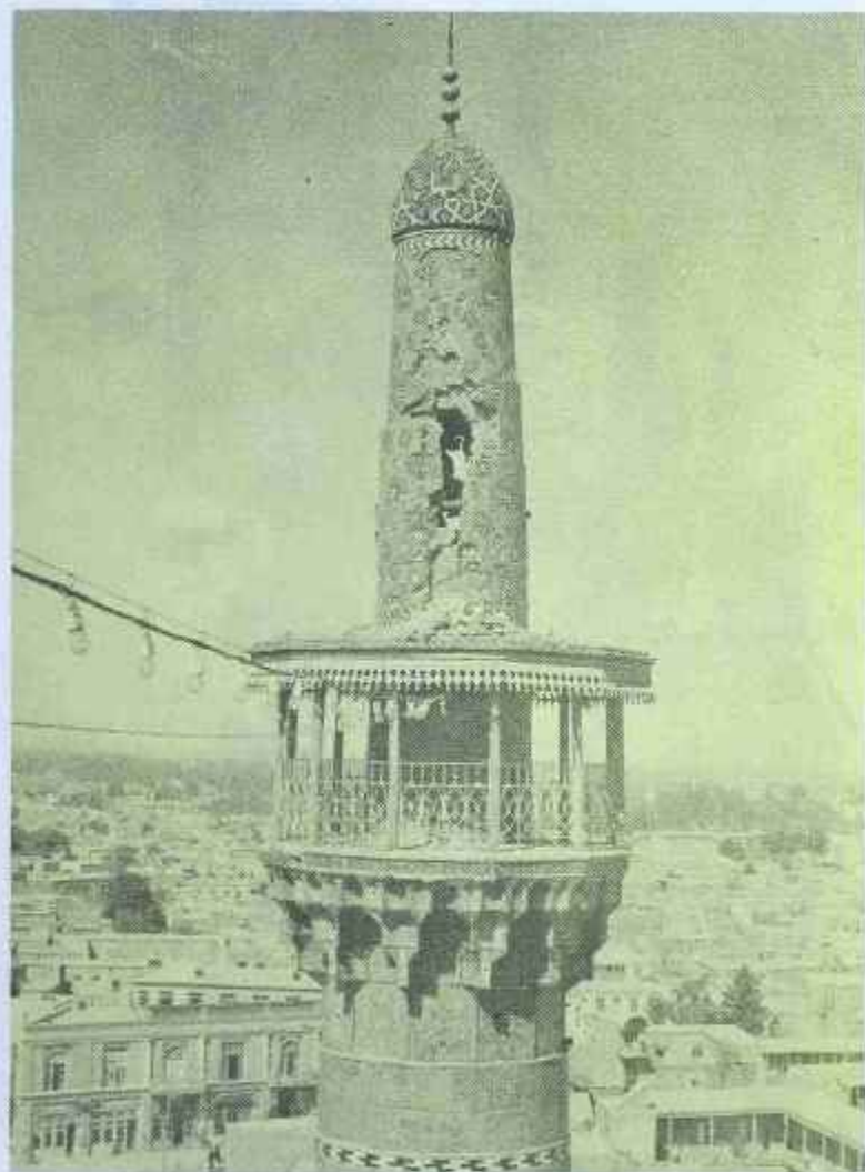
Due to an earth quake in 1315 (1936) the upper part of minaret of Gowhar Shad Mosque was ruined.
